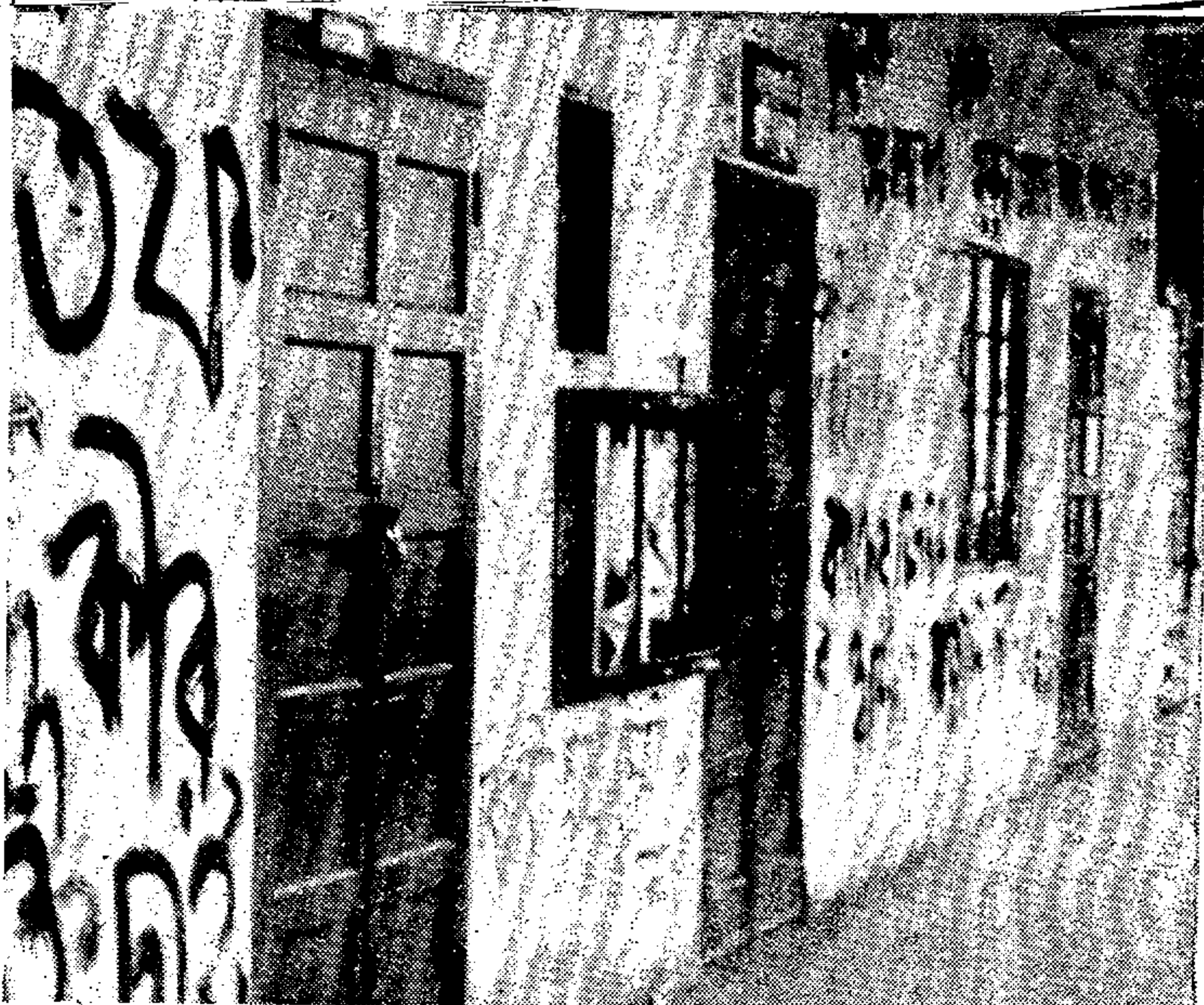
The gate of the Dhaka University Arts Faculty Building locked on Tuesday.—OBSERVER.
